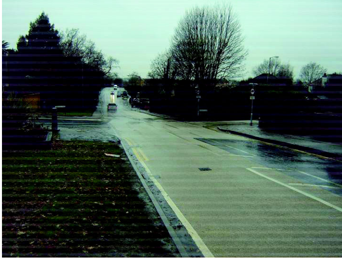
Image 3: Existing High Friction Surfacing at the Manor Road/Tomswood Road junction.
